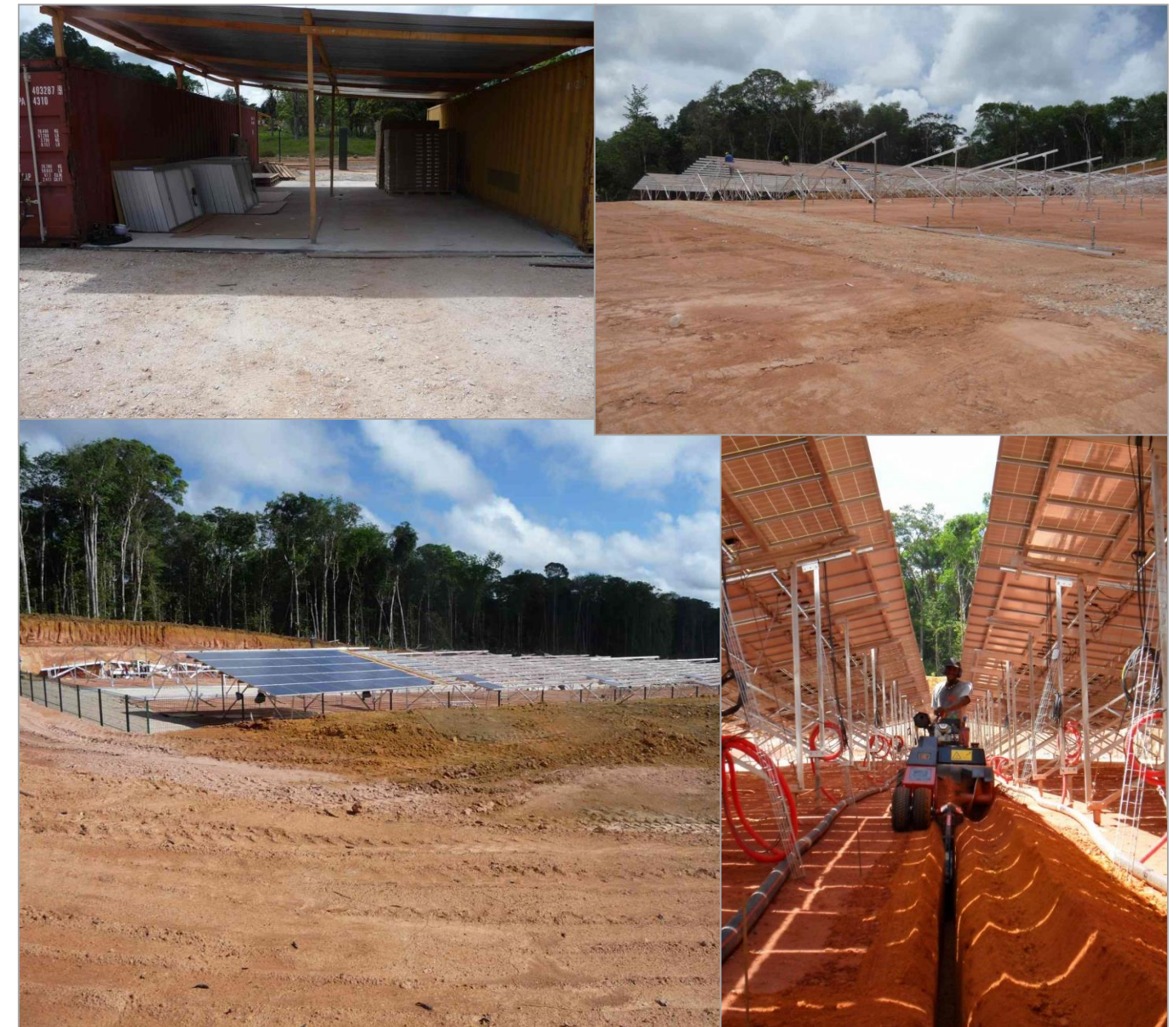
Figure 19 : Photos illustrant la phase chantier (source : VOLTALIA)
