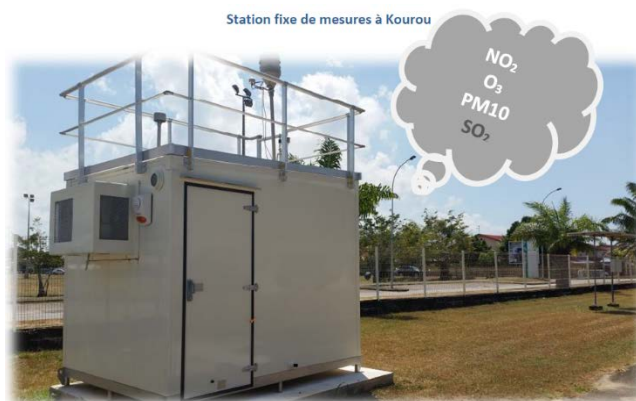
Figure 7 : Station de surveillance BRADY à Kourou, ORA 2017
