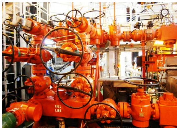
Navire de forage, manifolds - STENA ICEMAX
