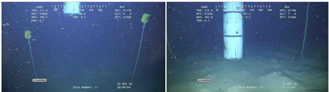
Figure 19: Descente du tube guide.
