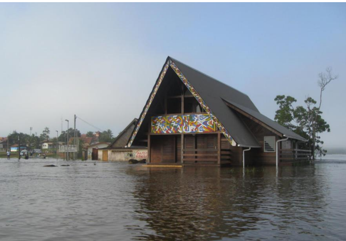
(Inondation Apatou 2008 - Source DEAL Guyane)
